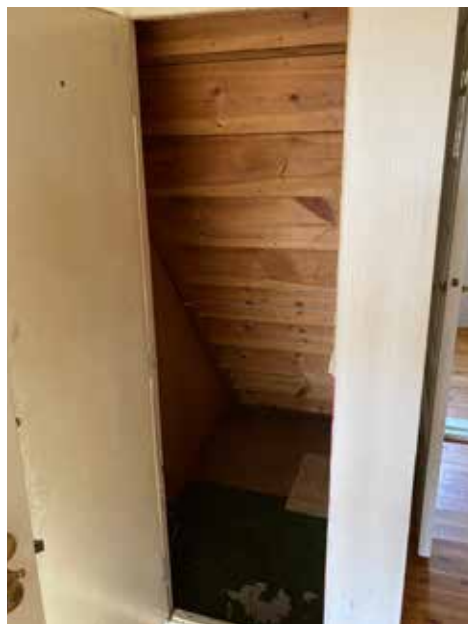
Bod i gang inn mot stove 2
