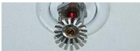
Figur 6 Sprinklerhode i himling
